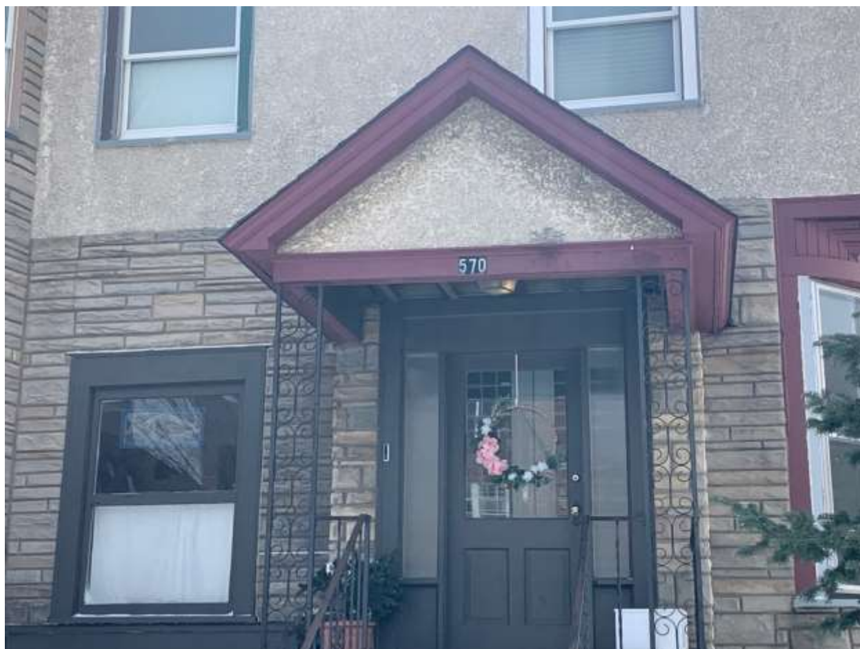
570 Portland Ave. Photo 3-17-23
